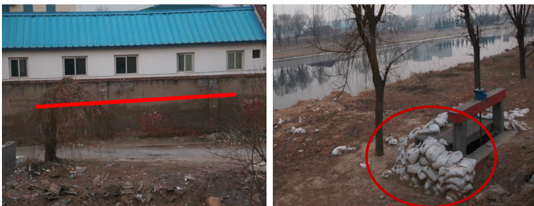
Figure 5 Aftermath of Grand Canal Forest Park in Tongzhou Dist.; the red line denotes the height of the maximum flow during the flooding period (Source: photos were taken of the Grand Canal Forest Park on the afternoon of Dec.11 by author)
