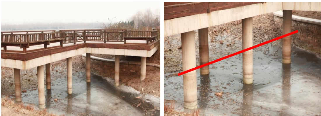
Figure 5 Aftermath of Grand Canal Forest Park in Tongzhou Dist.; the red line denotes the height of the maximum flow during the flooding period (Source: photos were taken of the Grand Canal Forest Park on the afternoon of Dec.11 by author)
